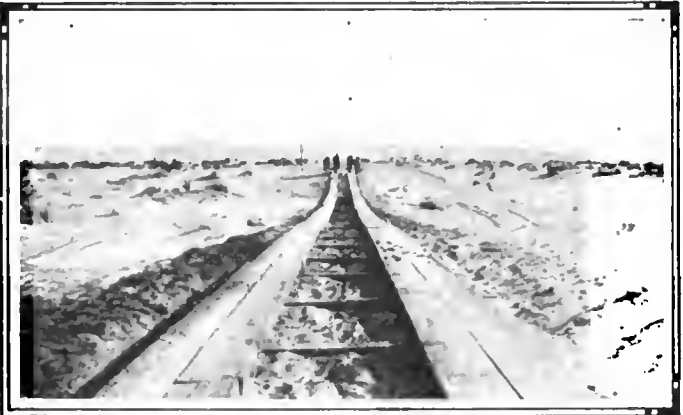
How the lumber road appeared just after boards were laid on the ties and before the road bed had been filled in
